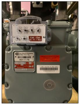
Honeywell American Meter AC-250 Class Gas Meter
